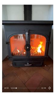
Main vent 75% closed. Door still ajar. Fire already established with smoke exhausting well from chamber.
